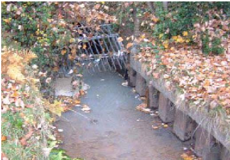
Fig V: Mouth of the railway culvert (Taken by Austin, S)
